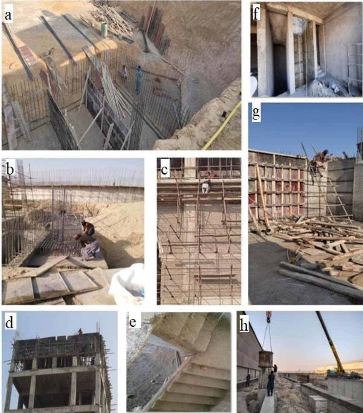
Figure 1: Safety violations observed at various construction sites including Poor Site Layout (a), Poor site layout (b),
