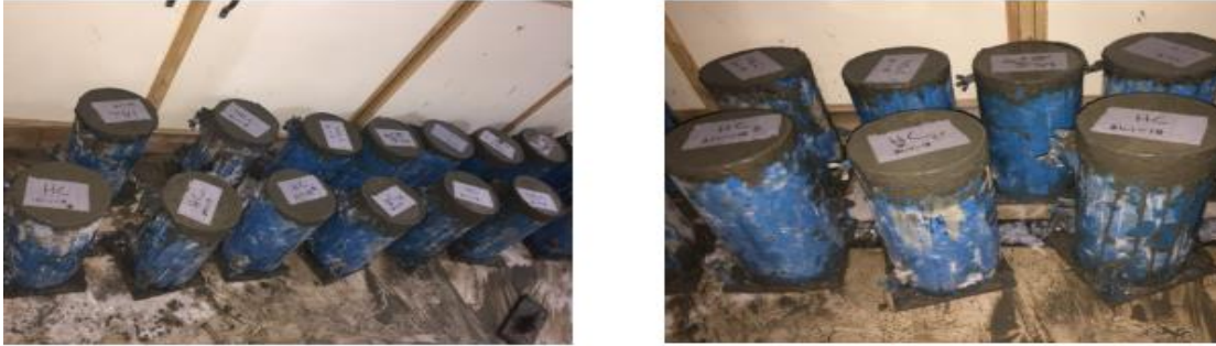
Figure 14 Casting and Curing of Concrete Sample
